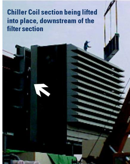
**Chiller Coil section being lifted into place, downstream of the filter section**
